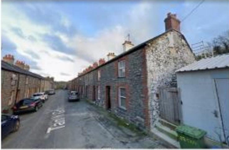
Photograph | Typical terrace housing located to the North
